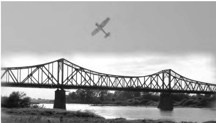
Fig. 1.1. Engineering structures (photographed by M. Rucka)
